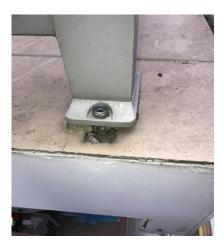
Above: Improper water proofing around balustrade fixing providing areas for water ingress to structural elements.
