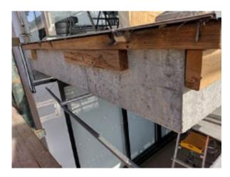
Above: Balustrade posts half supported on concrete slab and half supported on timber screwed into the side of the slab.
