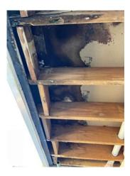
Above: Underside of balcony; substrate with significant rot from water and timber joists showing rot.
