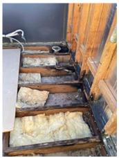
Above: Upper level balcony; tiling removed to show rotten timber to balcony structure, and
