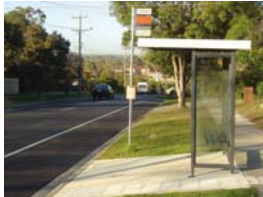
Figure 25: Continuous accessible pedestrian path
