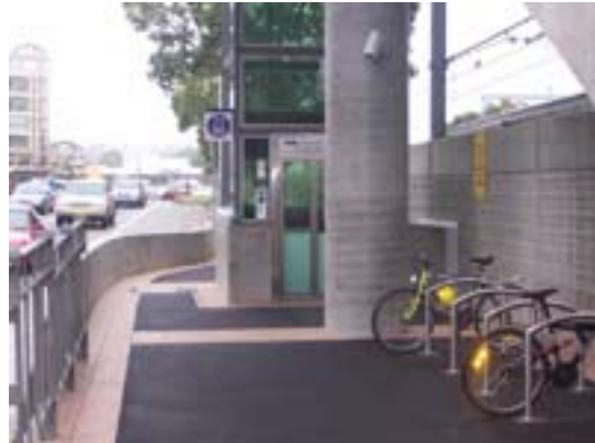
Figure 39: Transport Interchange Epping - NSW
