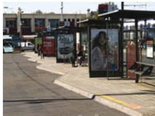
Figure 41: Sawtooth bus bays
