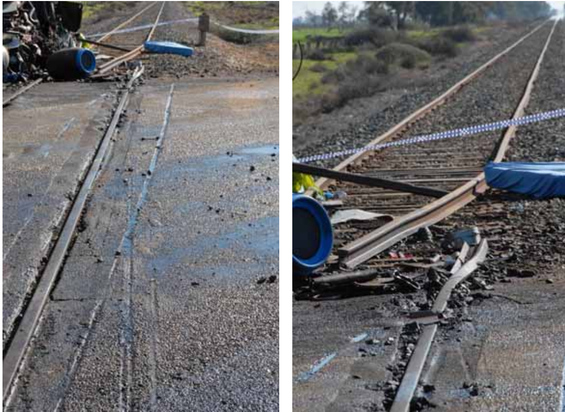
Figure 6. Looking towards Swan Hill, derailment marks (left) and broken rail (right)
