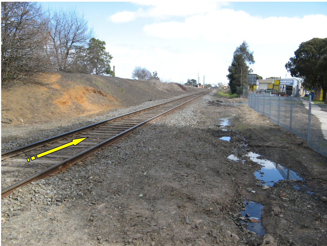
Figure 3: View of the Down approach to Queen Street, looking towards Warrnambool.
