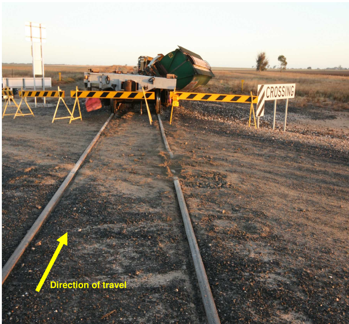
Figure 1 – Mellis Road level crossing and the derailed wagons in the background
