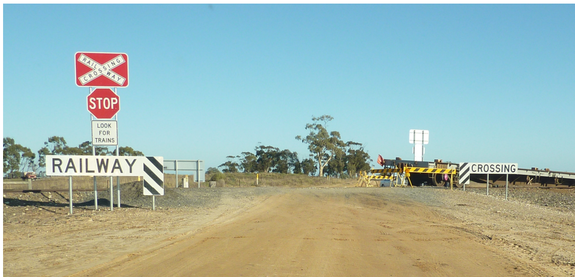
Figure 3 - Mellis Road level crossing
