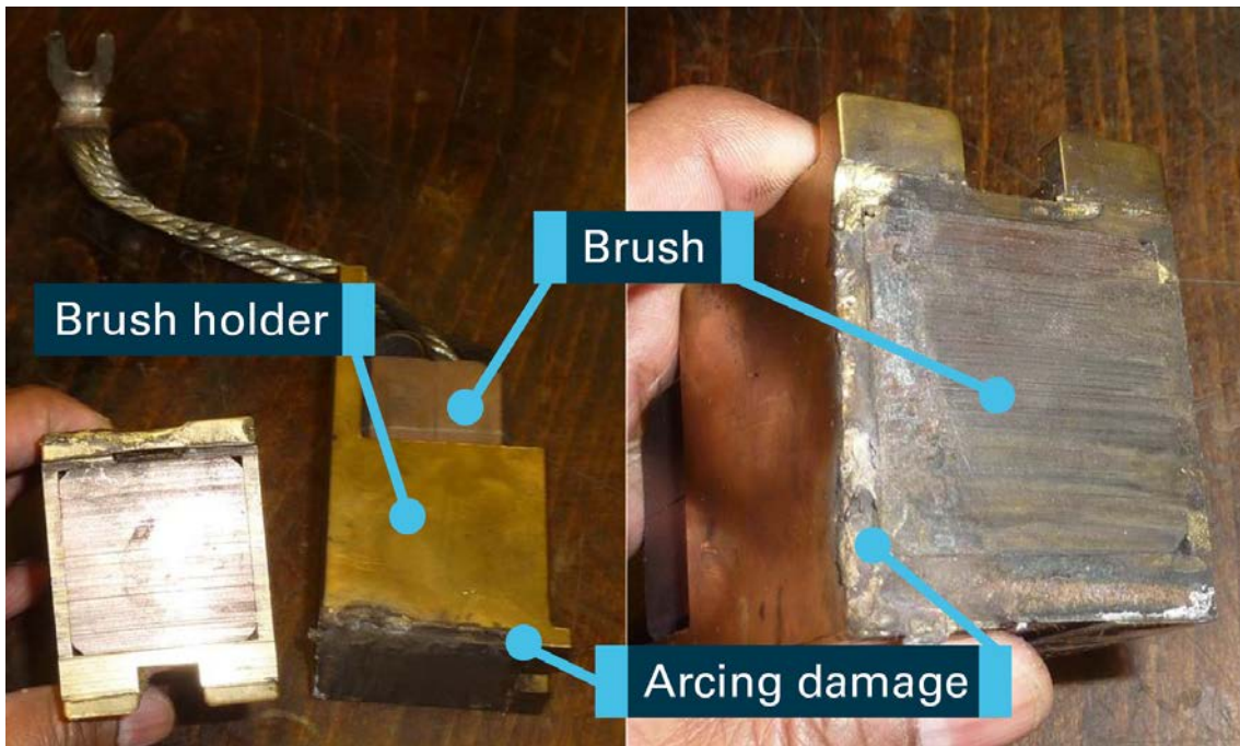
Figure 7: Arcing damage to brush holders
