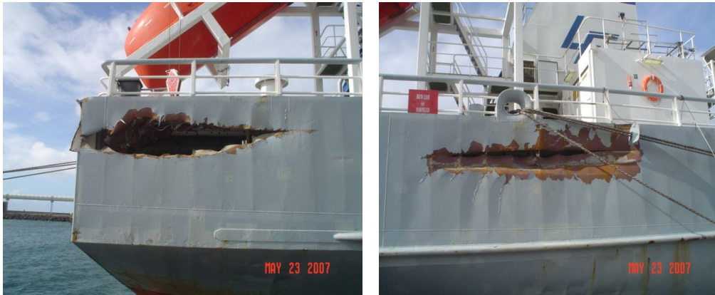
Figure 2. MV Bison Express ship side damage.
