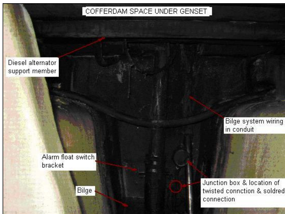
Figure 8 - Cofferdam space under Genset
