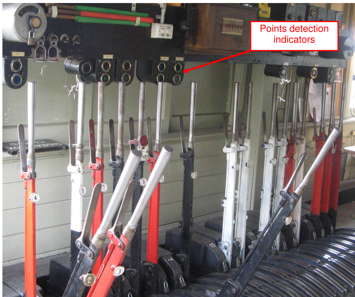
Figure 4 Kensington signalbox – lever frame.
