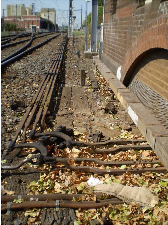
Figure 5 Kensington signalbox – point rodding.
