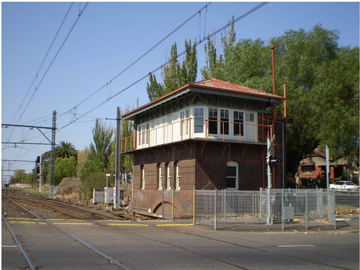
Figure 3 Kensington signalbox – February 2009.
