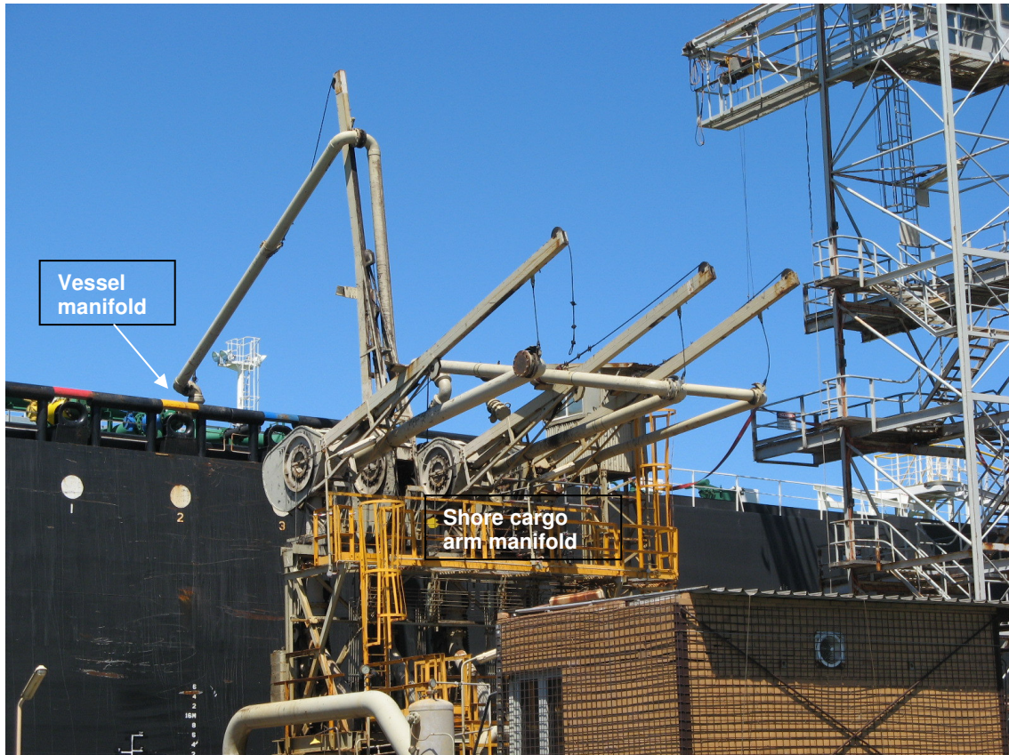
Figure 2 – Shore cargo arm connected to vessel's manifold (The vessel pictured is not Leyte Spirit)
