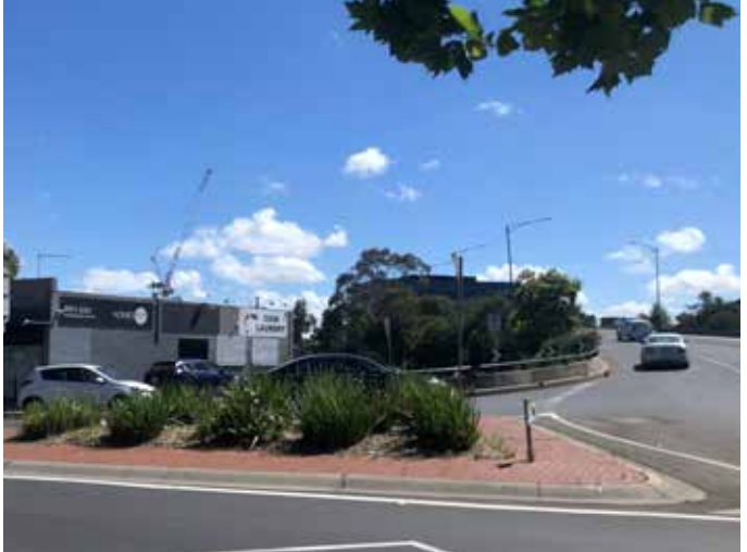
Existing view of Hampshire Road Bridge and the approach to the roundabout from Sun Crescent.
