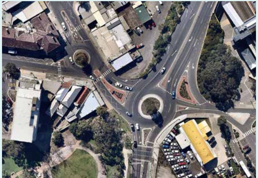
The current roundabout at the western end of Hampshire Road bridge.
