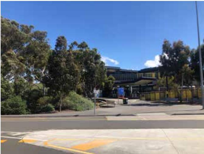
Existing view looking east to the station entrance on the western side of the station.
