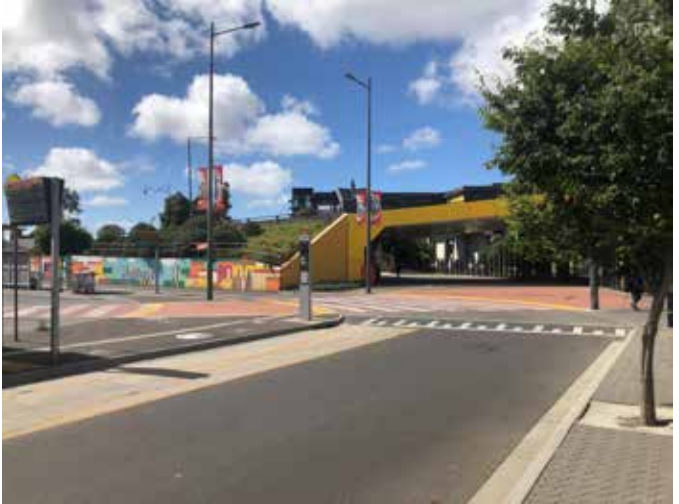
Existing view looking south to the station entrance beyond the Hampshire Road bridge underpass.
