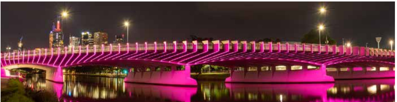
New feature lighting on the upgraded Swan Street Bridge in Melbourne.
