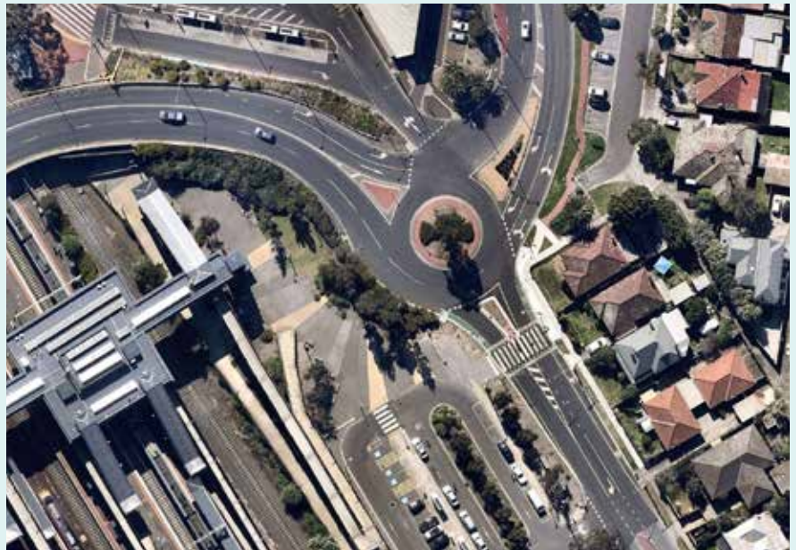
The current roundabout at the eastern end of Hampshire Road bridge.
