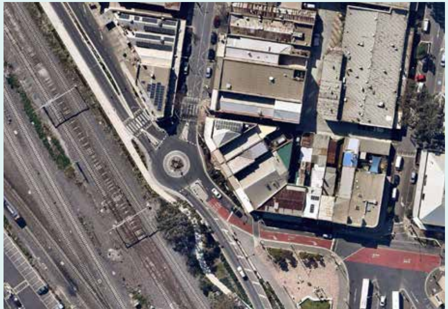
The current roundabout at the junction of Harvester Road / Hampshire Road / Dickson Street.
