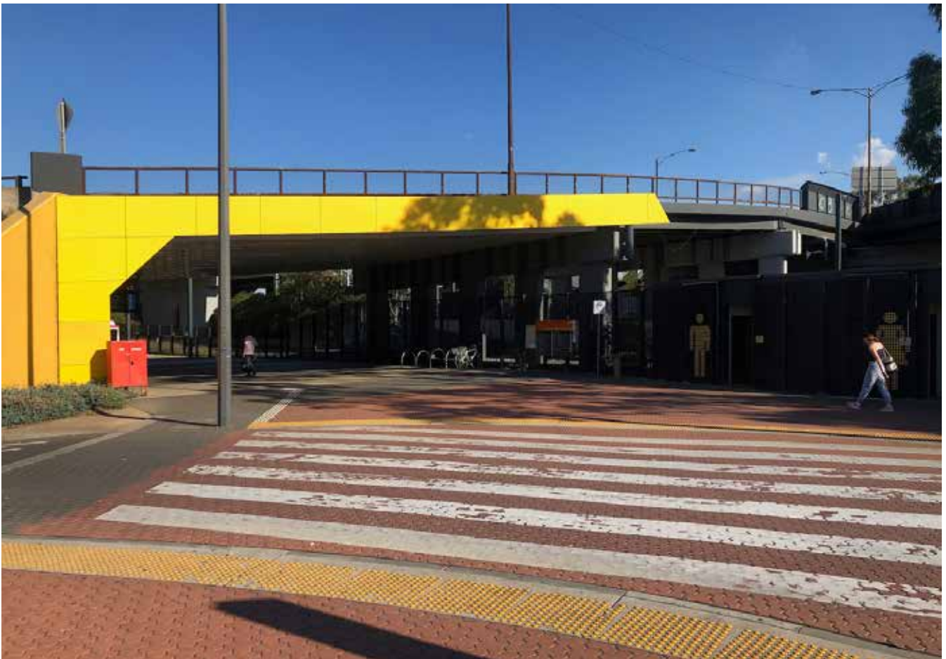
View of how the current entrance to Sunshine Station on the eastern side is obscured by Hampshire Road bridge.
