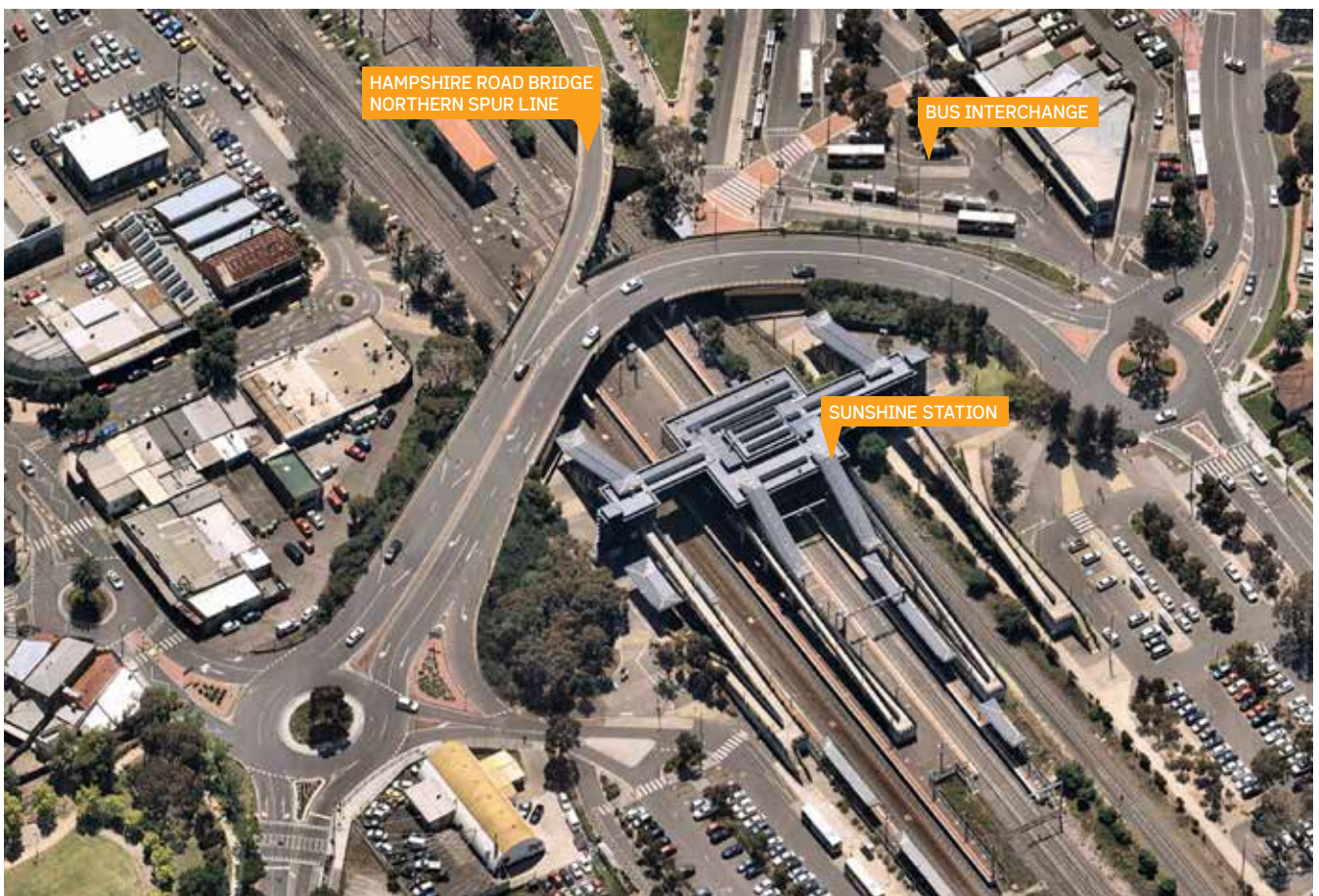
View of Hampshire Road bridge, looking north towards central Sunshine.
