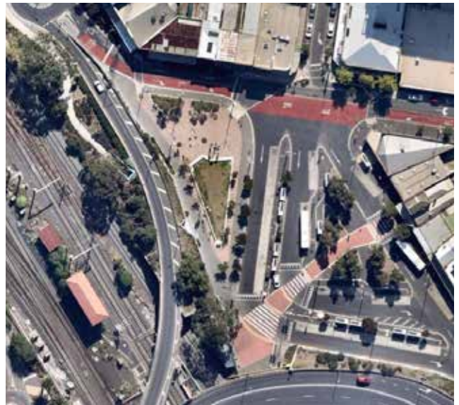
Aerial of the existing space.
