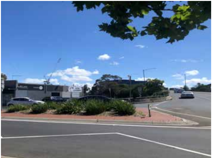
Existing view of Hampshire Road Bridge and the approach to the roundabout from Sun Crescent.
