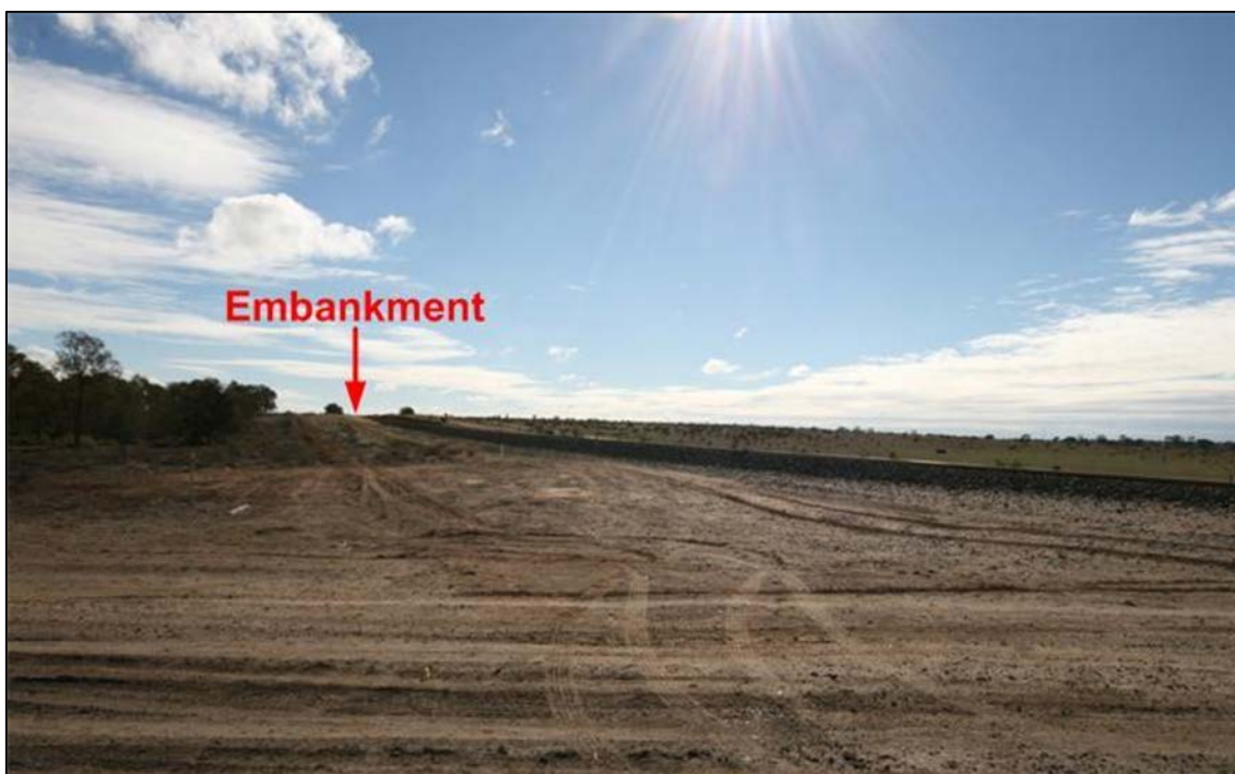
Figure 8: View looking north, about 20 m from the crossing
