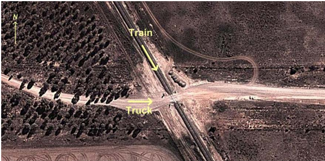
Figure 5: Aerial view of B. McCann Road level crossing.
