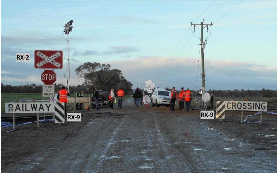
The image is a close-up view of the crossing showing the level crossing signage. Source: Chief Investigator, Transport Safety (Vic)
