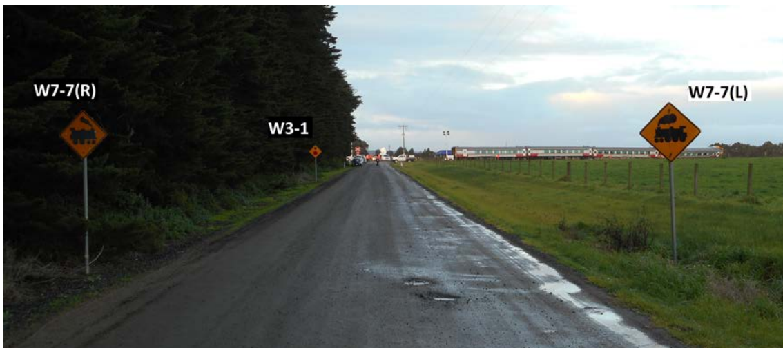
The image shows the view for a road-user about 250 m from the crossing. The Railway Crossing Ahead signs (W7-7) are in the foreground, and the Stop Sign Ahead sign (W3-1) beyond. Source: Chief Investigator, Transport Safety (Vic)
