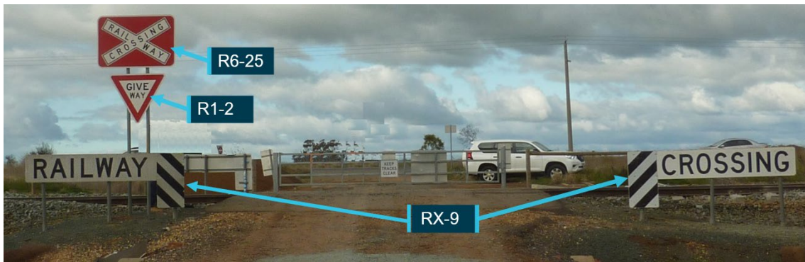
Figure 6: Holmes Road level crossing access from west of the rail track
