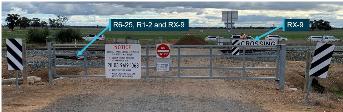
Figure 5: Holmes Road level crossing access from east of the rail track
