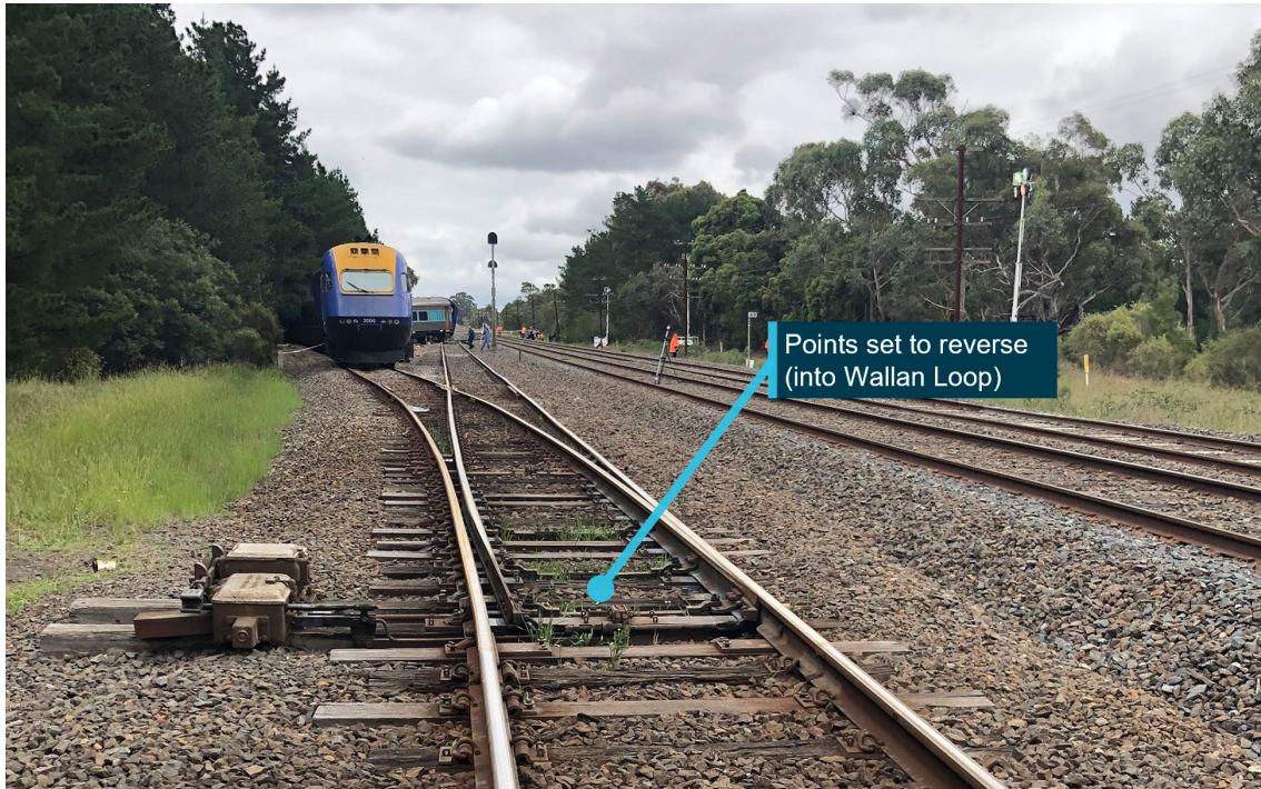
Figure 14: No. 7 points at the northern entrance to Wallan Loop set to reverse
