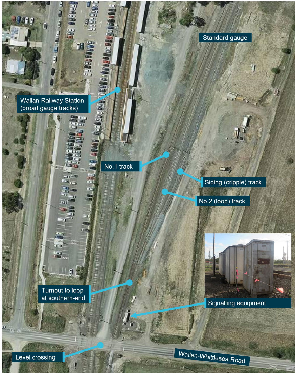
Figure 9: Aerial view of Wallan–Whittlesea Road level crossing and surrounds
