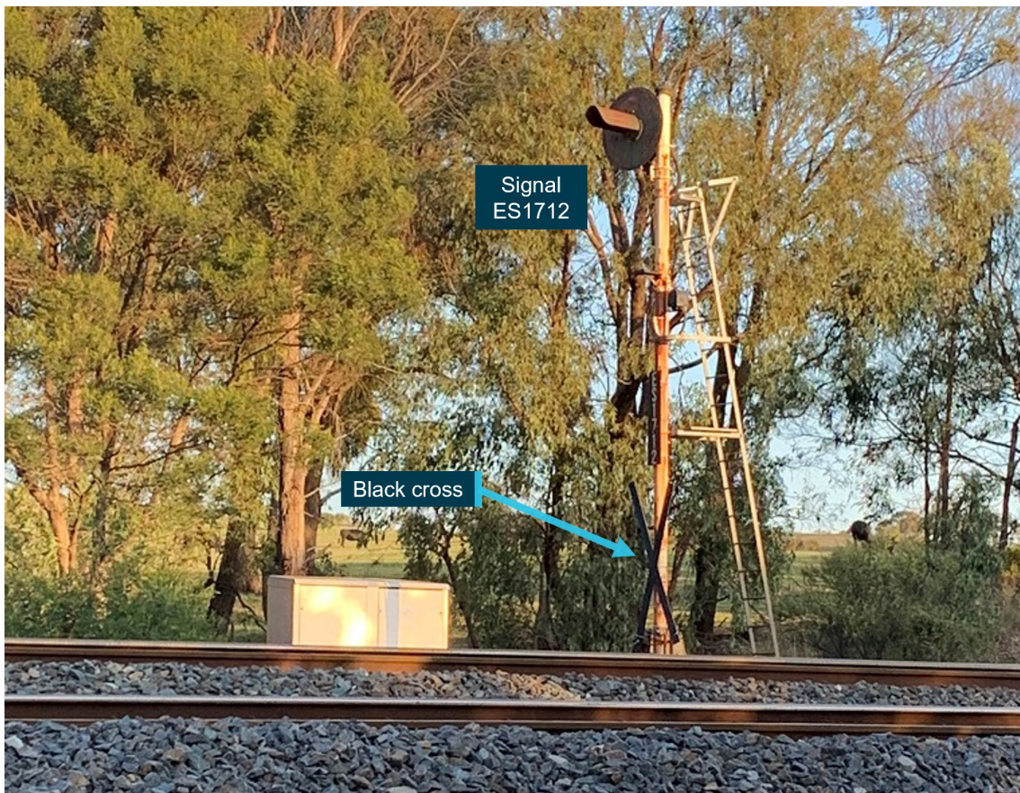
Figure 10: Signal ES1712 following derailment, non-operational and with cross affixed
