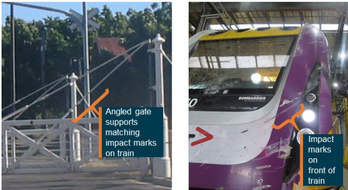
Figure 3: Impact damage to the front of train 8185, car 1270
