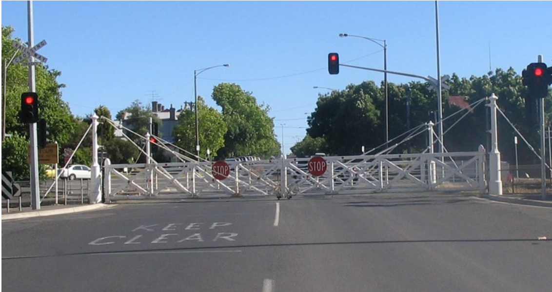
Figure 9: Level crossing gates at Lydiard Street North, approaching from the south
