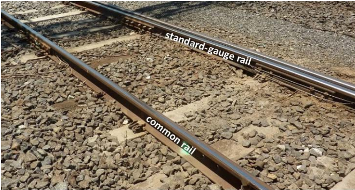
Figure 4: Track construction at point of derailment
