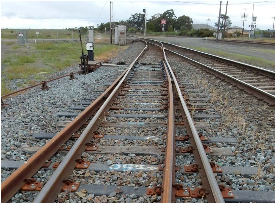
Figure 18: The derailment location after rectification works
