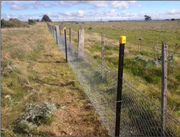
Plate 7. Pest-fauna proof fence along the northern boundary of the offset site (July 2014)
