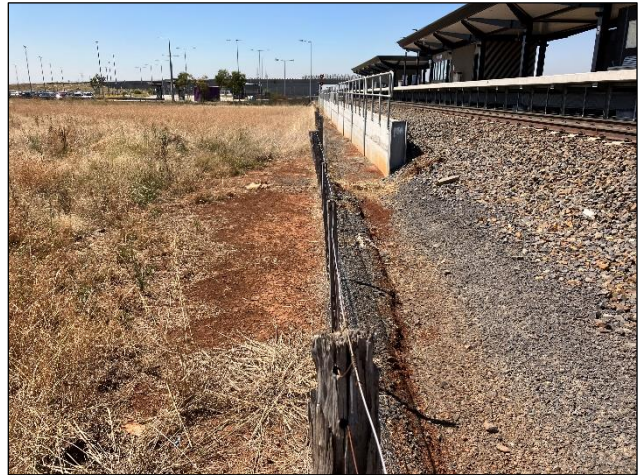
Plate 26. Area west of the drain showing little rubbish and debris likely to flow into and block the drain (Ecology and Heritage Partners 9/02/2023).
