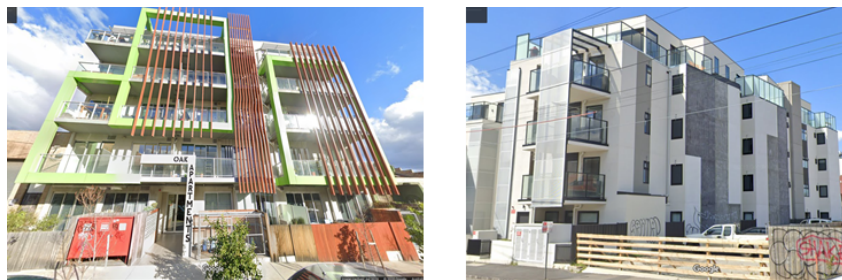
Figure 5.3: Buildings with combustible cladding that differ principally in the RAT egress provisions rating
