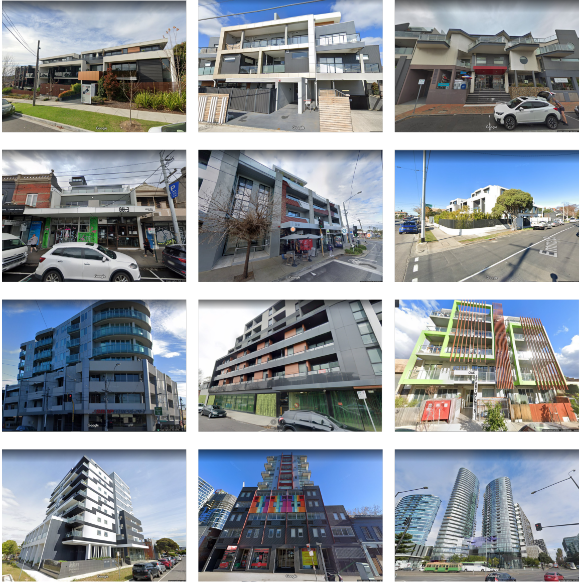
Figure 3.4: A selection of Melbourne metropolitan Residential Class 2 buildings with combustible cladding (all images copyright Google)
