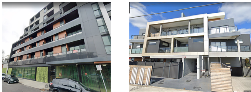
Figure 5.2: Buildings with combustible cladding that differ principally in the number of apartments and height
