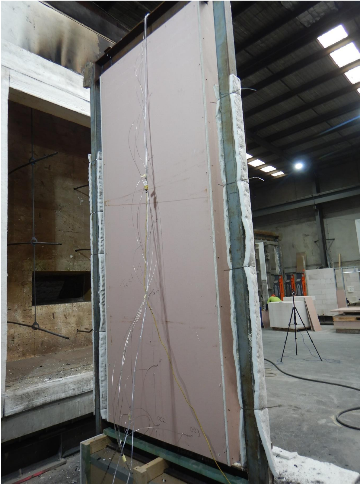
Figure 26 The specimen after the test – unexposed side.
