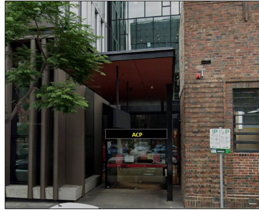
Figure 23: ACP panel at the head of the exit door.
