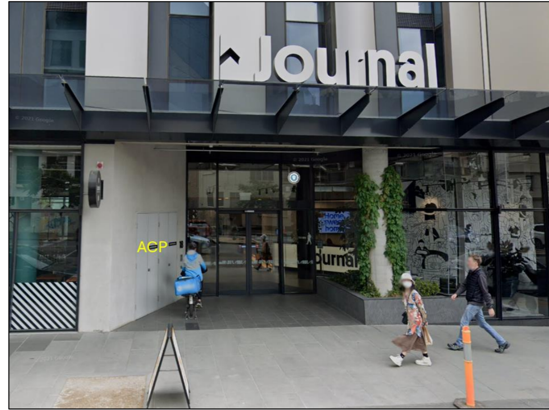
Figure 27: ACP cladding to service doors on the left of the exit. No sprinkler protection to exit.
