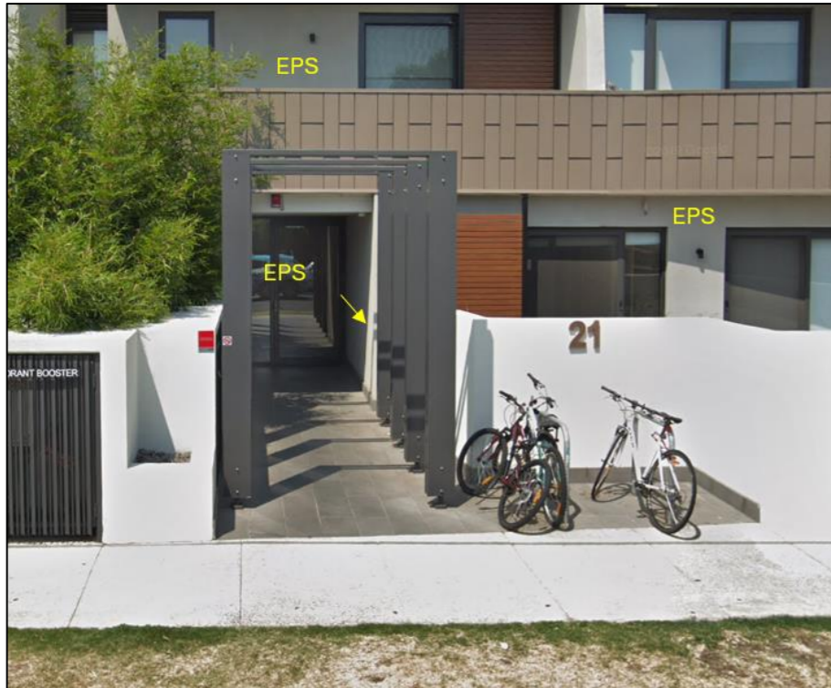
Figure 28: EPS cladding on SOUs above and below the exit. EPS to cladding around the exit. Sprinkler protection to SOUs.
