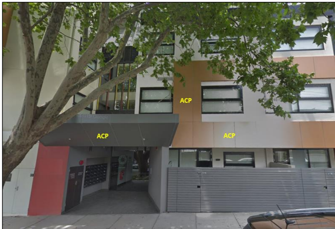
Figure 44: ACP canopy and soffit to entry alcove. ACP on front facade adjacent window openings. Sprinkler protected internally and within entry alcove.
