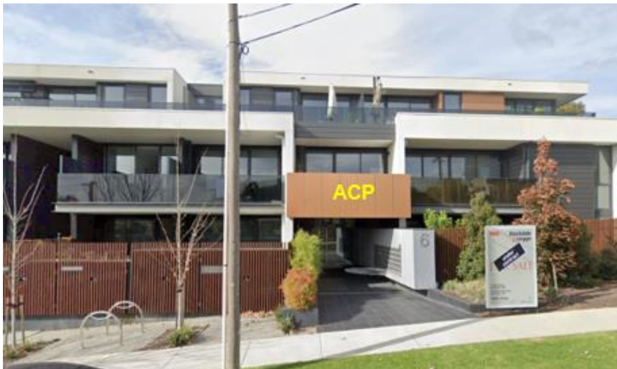
Figure 11: ACP cladding at the balcony balustrade of the building
