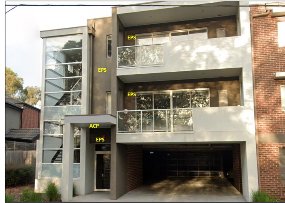
Figure 43: Element of EPS above the door. ACP on the soffit and face of the canopy. Sprinkler protection to SOUs.
