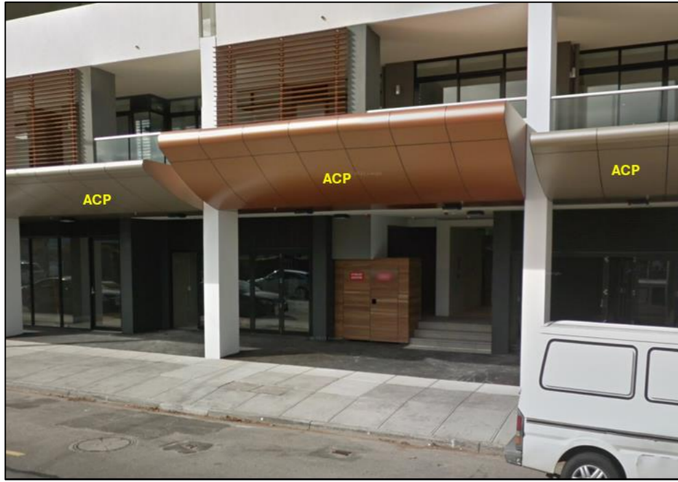
Figure 38: ACP awning projection forward of the external wall at GFL. No sprinkler protection to SOUs.
