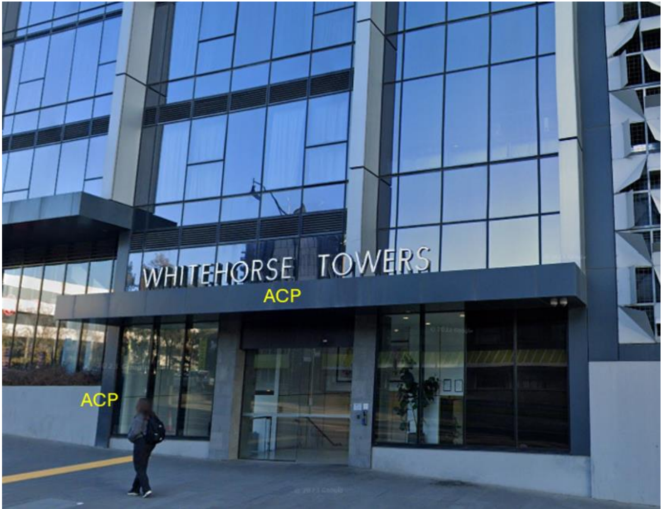
Figure 13: Large amounts of ACP around exit area
