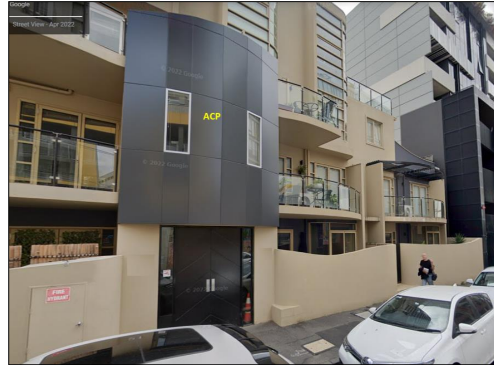
Figure 35: ACP to cladding above exit, no sprinkler protection to SOUs or exit.
