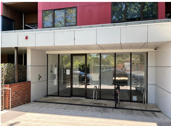
Figure 6: The ACP element extending to ground level creates a risk of benign fire ignition resulting in a problematic fire
