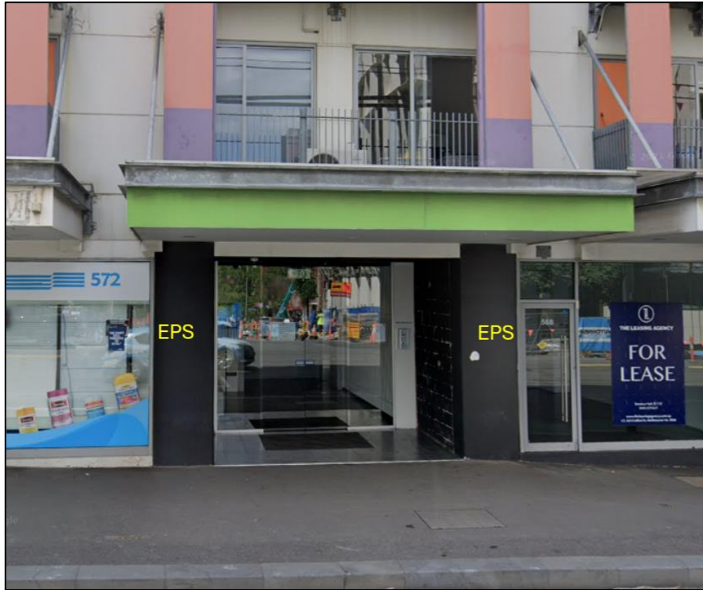
Figure 26: Single exit building, EPS to either side of the exit. No sprinkler protection.
