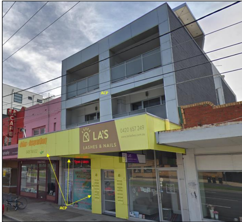
Figure 34: ACP cladding to canopy above and to either side of exit, no sprinkler protection to SOU or exit.
