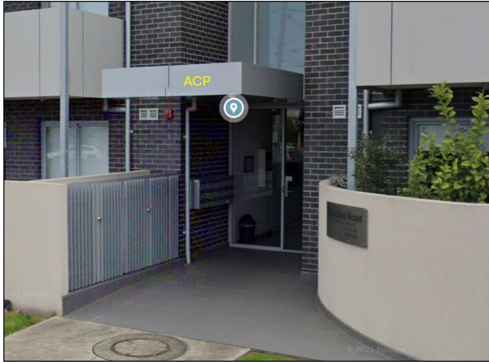
Figure 14: Single exit, ACP to canopy fascia. Soffit panels are non-combustible material, non-sprinklered exit.
