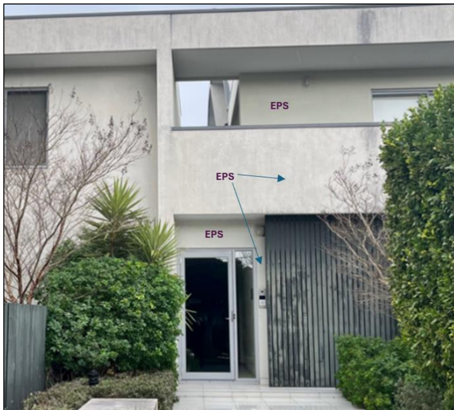
Figure 36: EPS on L1 and L2 on external walls over the main entry/exit – no sprinkler protection. SOU to the right of the exit.
