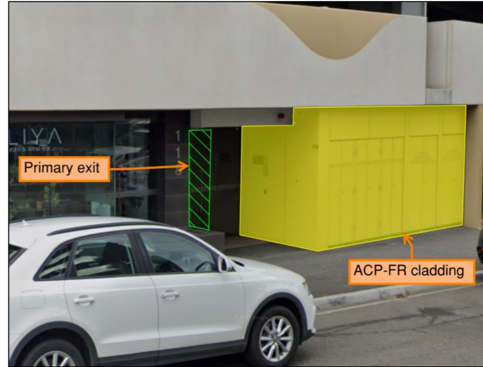
Figure 39: ACP-FR panels on the right side of the primary exit.
