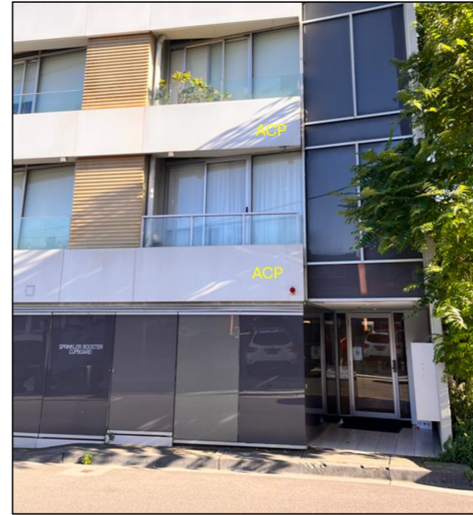
Figure 15: Single exit, ACP cladding to spandrel panels to the left of the exit, non-combustible material around the exit. Non sprinklered exit/building.
