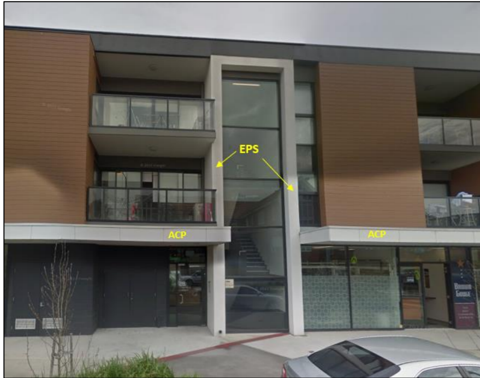
Figure 30: EPS panels above the exit and ACP to canopy face – sprinkler protection to SOUs.
