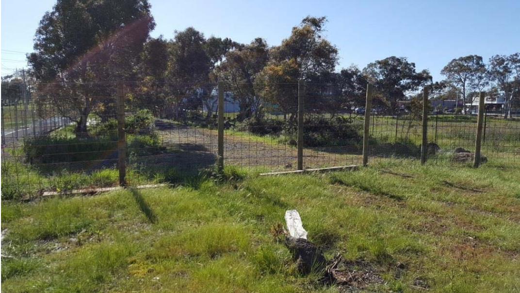
Figure 3. New fence section, installed over past vandal access point
