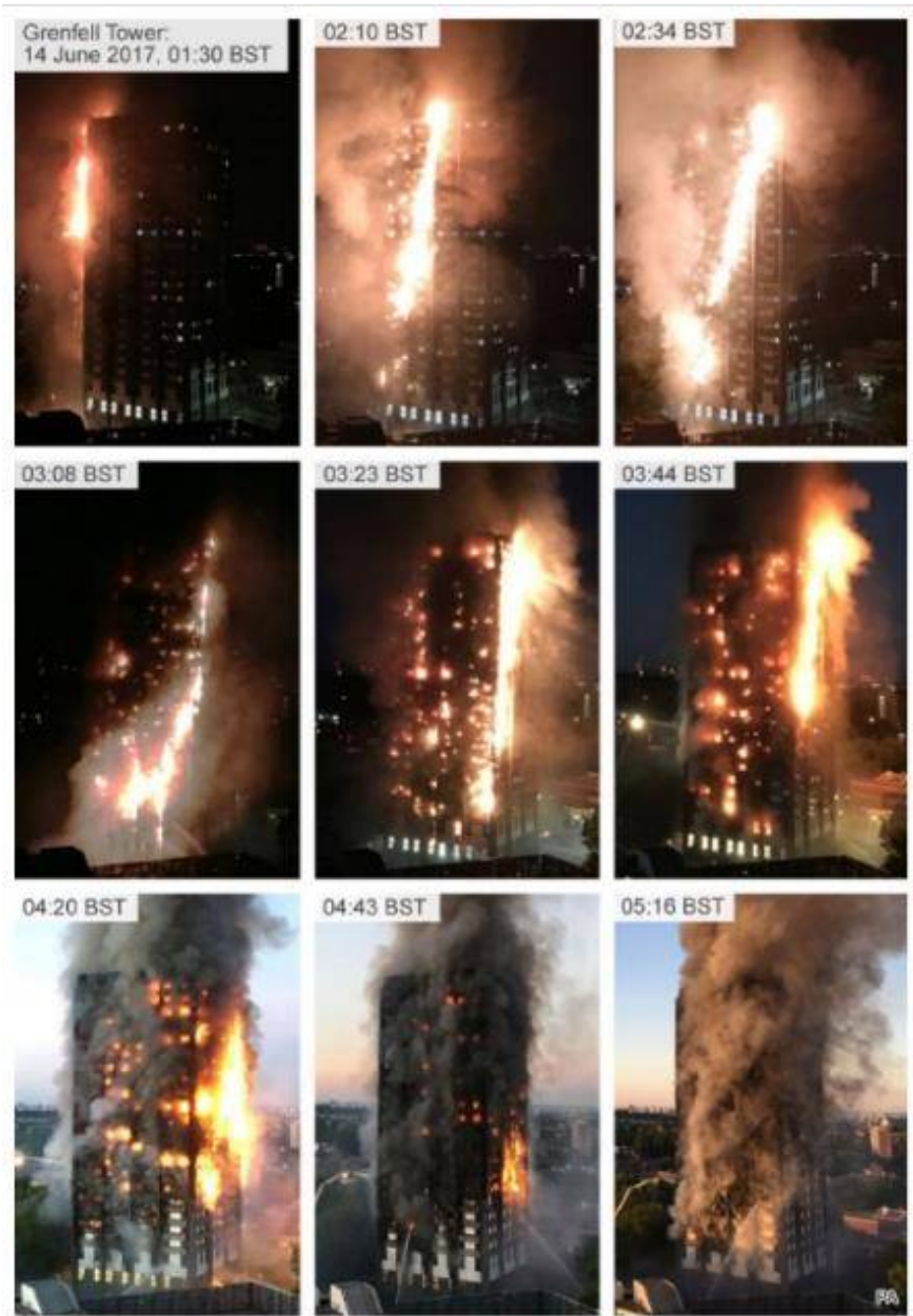
Figure 53. Grenfell tower fire spread (image from BBC News [64] )
