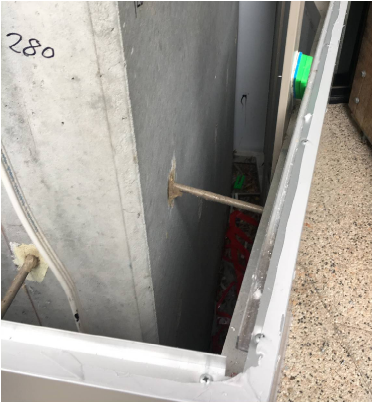
Figure 3: Cassette mount installation onto column (Photo by CSIRO)
