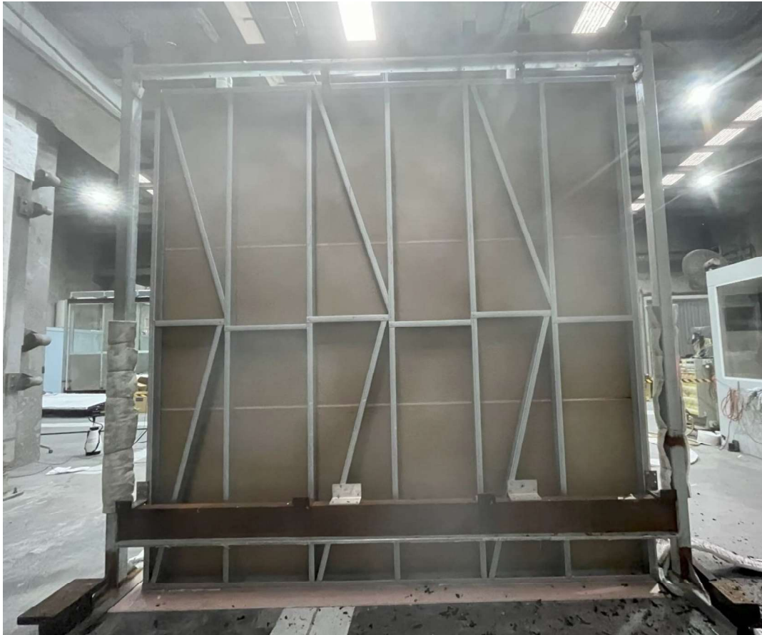
Figure 32 The unexposed side of the specimen at the end of test
