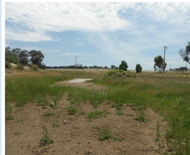
Plate 8: Dam 7 holding water at the time of the 2012 assessment
