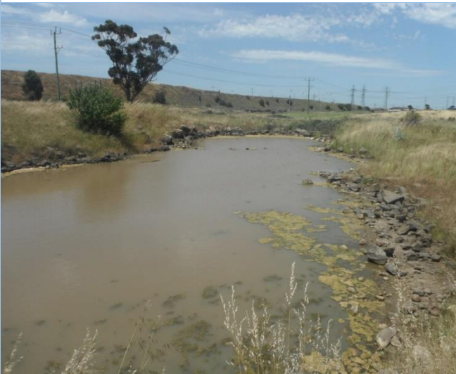
Plate 4: Dam 3 holding water at the time of the 2012 assessment
