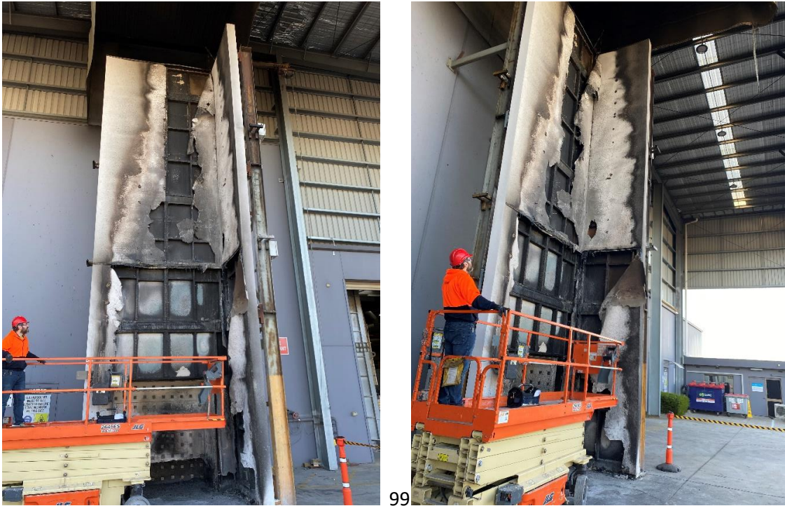
Figure 9. Post-test external rendered EPS wall system prior to any deconstruction. Main wall (left) wing wall (right)
