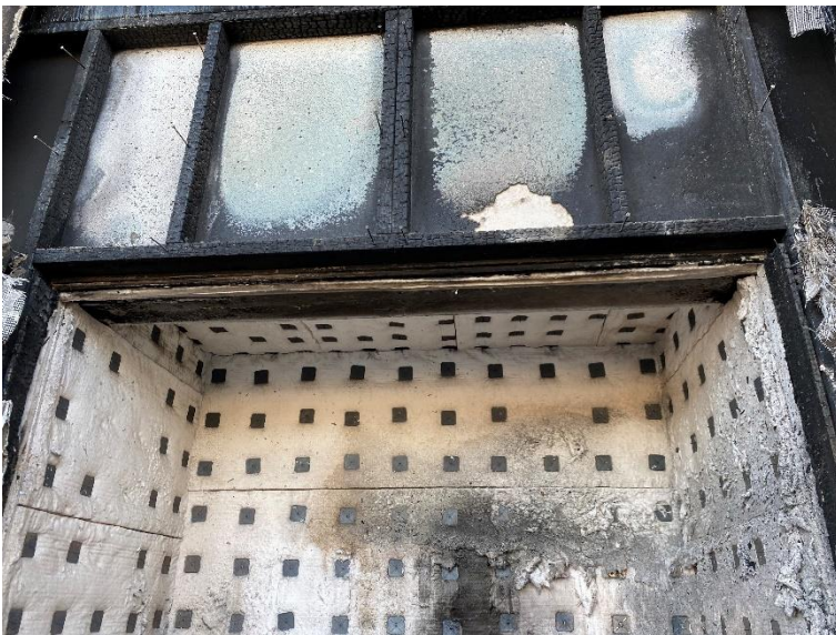
Figure 12. Post-test wall system close-up of combustion chamber opening and region of most heavily charred timber framing and heat effected plasterboard
