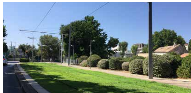
Figure 48. Permeable ground treatments along tram lines
