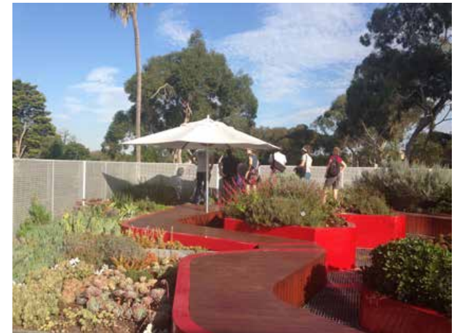
Figure 39. Integrated roof gardens, Burnley Campus, University of Melbourne
