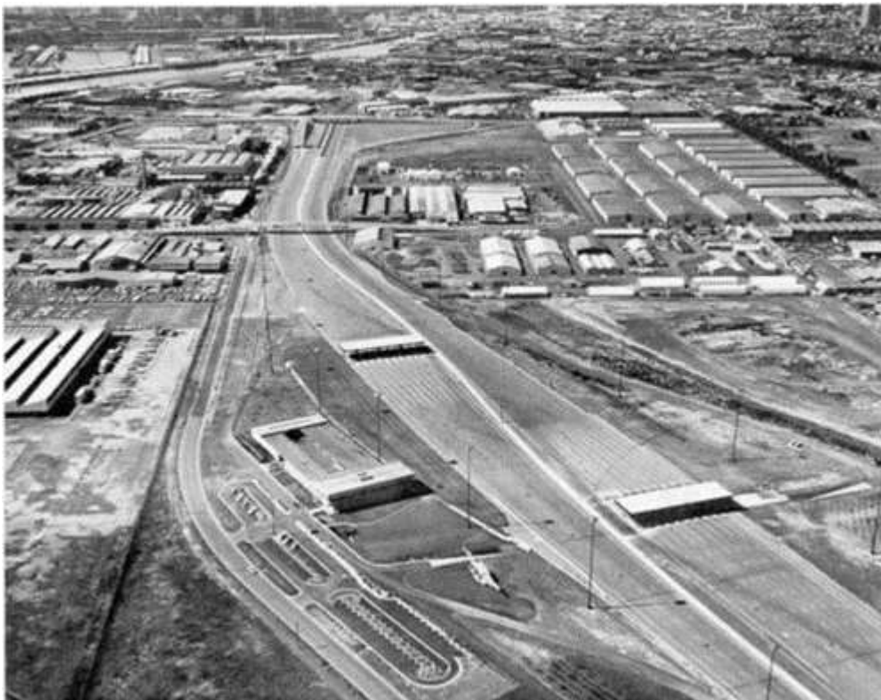
Figure 74: West Gate Bridge toll plaza looing east just prior to opening (Museum Victoria)
