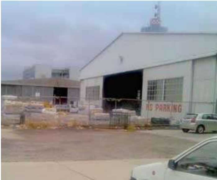
Figure 43: Butler Hangar at Fishermans Bend prior to relocation (National Trust)
