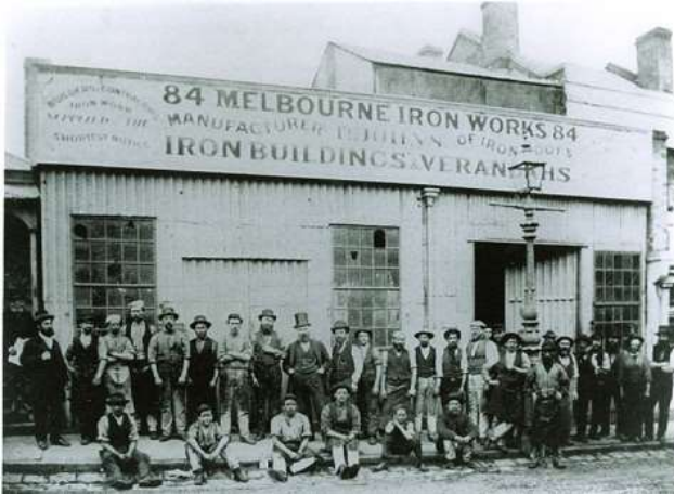
Figure 23: Beginnings of Johns & Waygood works (State Library Vic)
