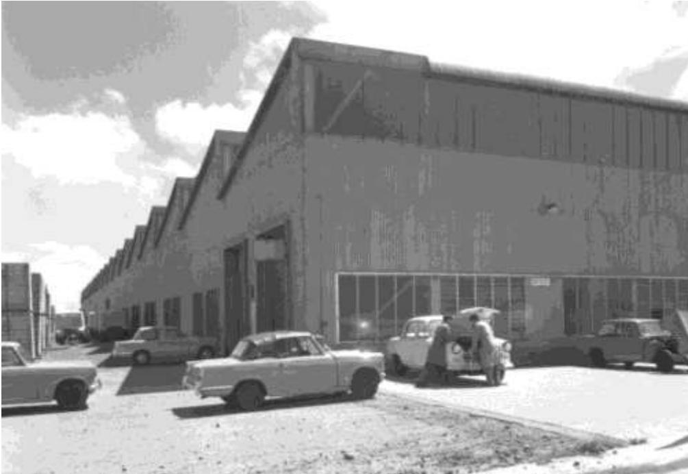
Figure 58: External view of the Standard Motor Products factory, 1962 142
