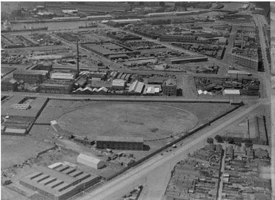
Figure 19: View to east from near Port Melbourne Football Ground showing Kitchen & Sons and warehousing/timber yards beyond.
