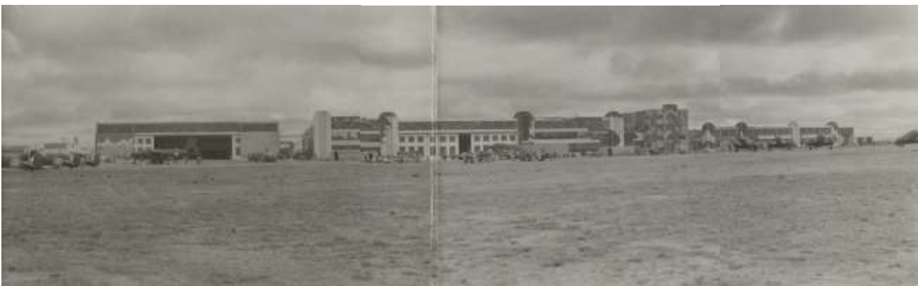
Figure 42: CAC from the south showing camouflage painted buildings 123
