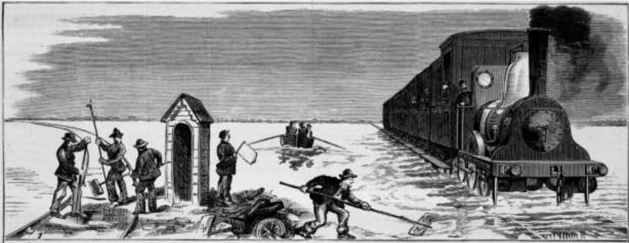
Figure 38: Floods along the Port Melbourne Line 108
