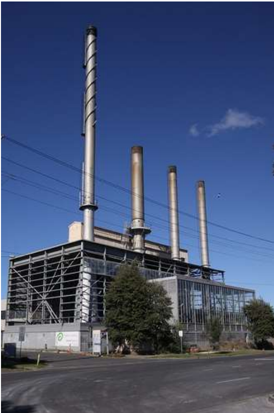
Figure 54: Demolished Holden Boiler House (Photo Wongm)
