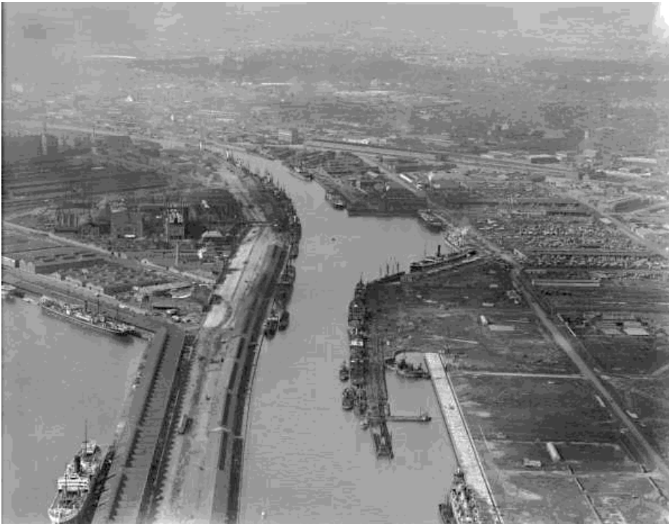
Figure 32: Yarra River and Port of Melbourne showing widening operations downstream of swinging basin. Between 1930 and 1948. 72
