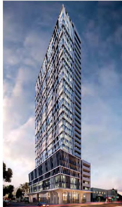
Figure 9: 89-103 Gladstone Street, South Melbourne. Source: Plus Architecture.
