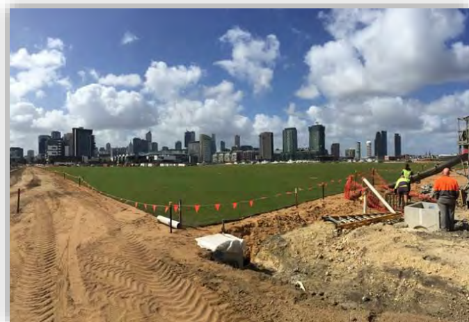
Figure 59: Ron Barassi Snr Park, Docklands with physical separate layer between site users and residual soil contamination (photograph by C. Wallis)
