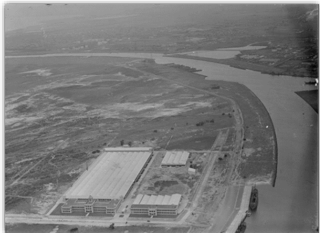
Figure 43: Original GMH factory, ca 1936, Pratt, CD & Airspy (1940), General Motors Holden (GMH) factory at Fishermans Bend, beside Yarra River, H91.160/258, Pictures Collection, State Library of Victoria
