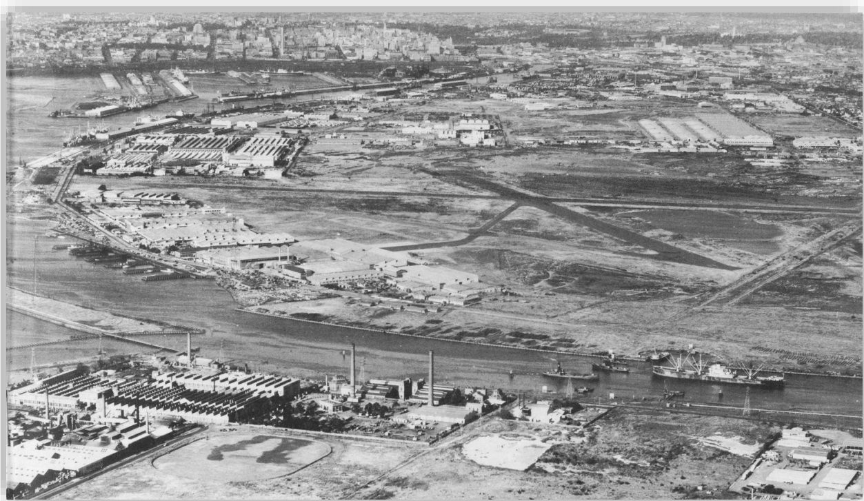
Figure 4: Photograph - Aerial View of Spotswood Pumping Station, Lower Yarra River & Fishermen's Bend, Victoria, circa 1954, Item MM 92390, Museum Victoria Collections (from MMBW Melbourne Metropolitan Planning Scheme report 1954, p.51).
