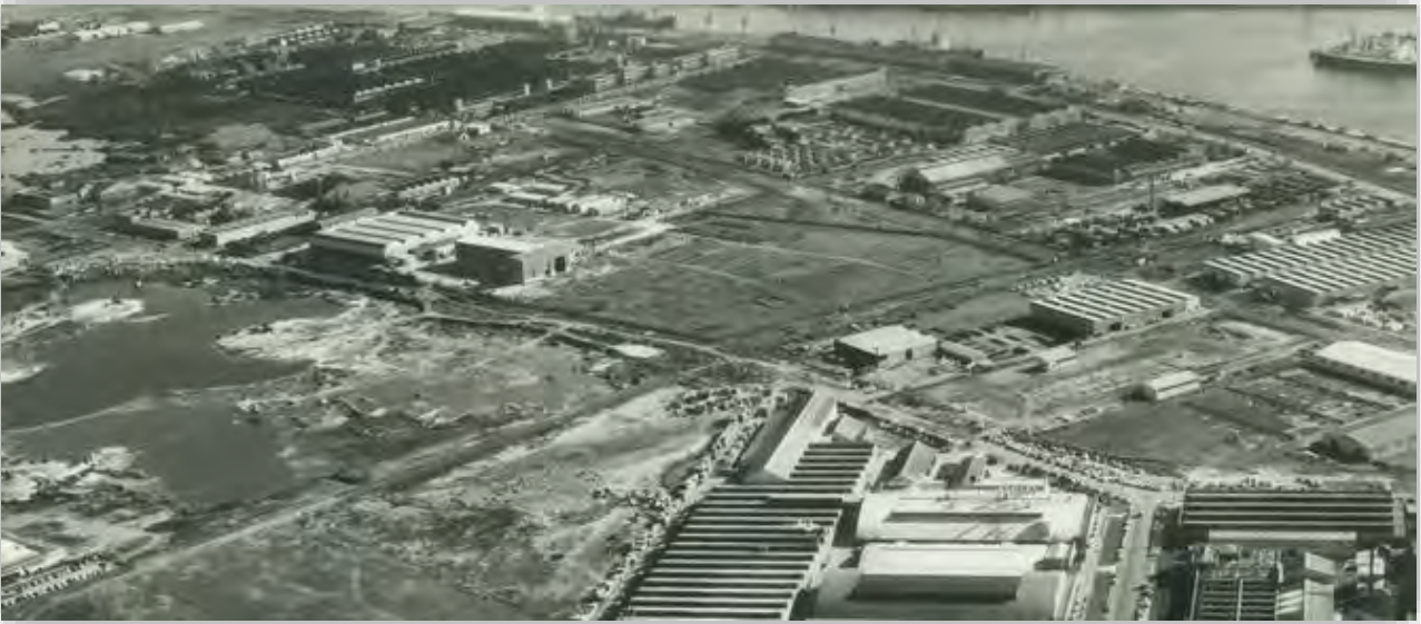
Figure 48: Pratt, CD & Airspy (1950), Aerial view of Fisherman's Bend, Image H2008.32/6. Pictures Collection State Library of Victoria, Note the former Melbourne Sand Works site in the bottom left corner and the recently SEC workshop under construction in the centre, Photo likely around early 1960s.
