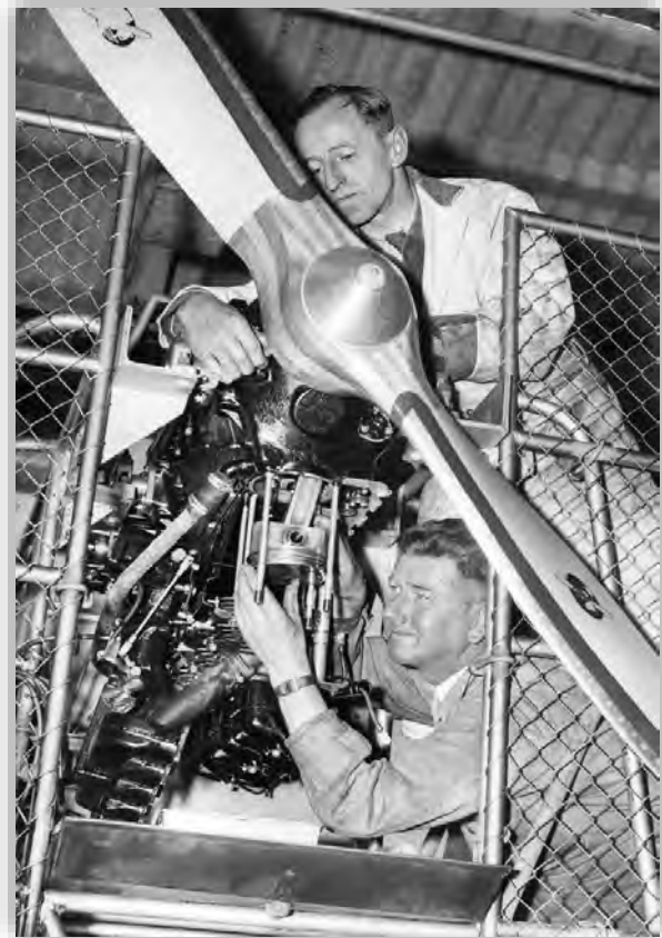
Figure 55: First Australian made Gypsy Moth goes out onto the test bench at General Motors – Holden's works at Fisherman's Bend. ca. 1940, Argus (Melbourne, Vic., H99.206/1951, Pictures Collection, State Library of Victoria
