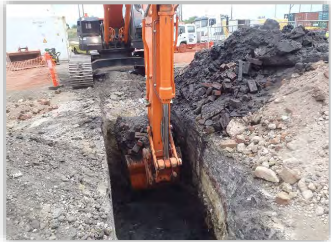
Figure 58: Example of investigation of former landfill. Dark soil impacted by waste oil (Photograph by P. Bentley).
