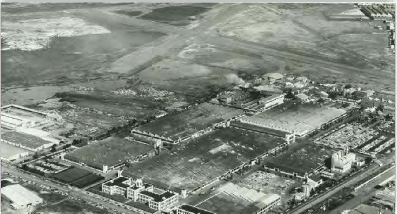
Figure 46: Pratt, CD & Airspy (1950), Aerial view of Fisherman's Bend, H2008.32/1, Pictures Collection State Library of Victoria. Note: Image likely taken around c1960.
