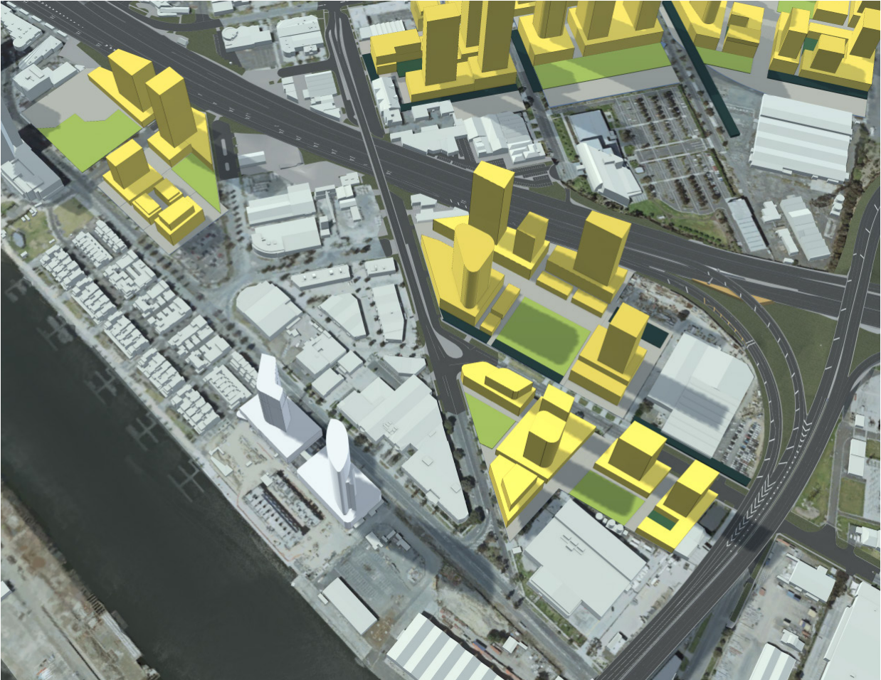
Figure 3 Lorimer perspective view - the application of the FAR together with all proposed building envelope controls support the delivery of the open space without loss of development yield on any site.
