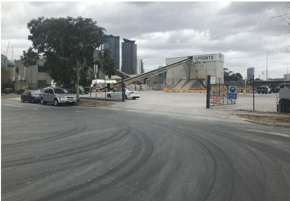
Figure 9 Barro concrete batching plant, abutting site to north and northwest
