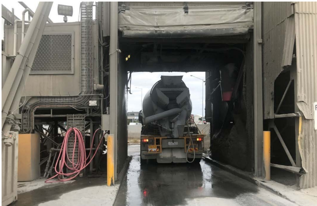
Figure 12 "Sock" where cement is loaded into vehicles
