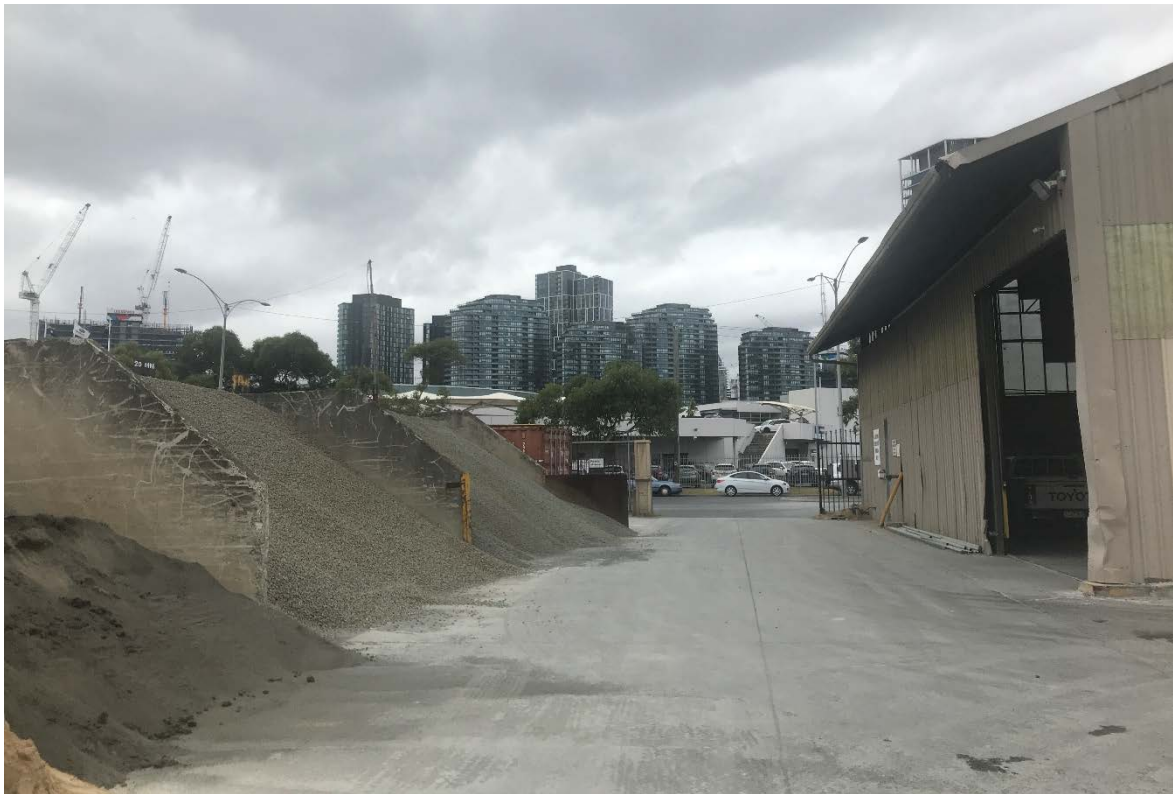
Figure 7 Material storage on the Hanson site
