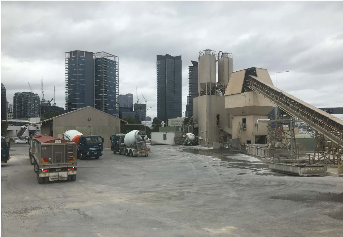
Figure 6 Existing conditions on the Hanson site (facing southeast)
