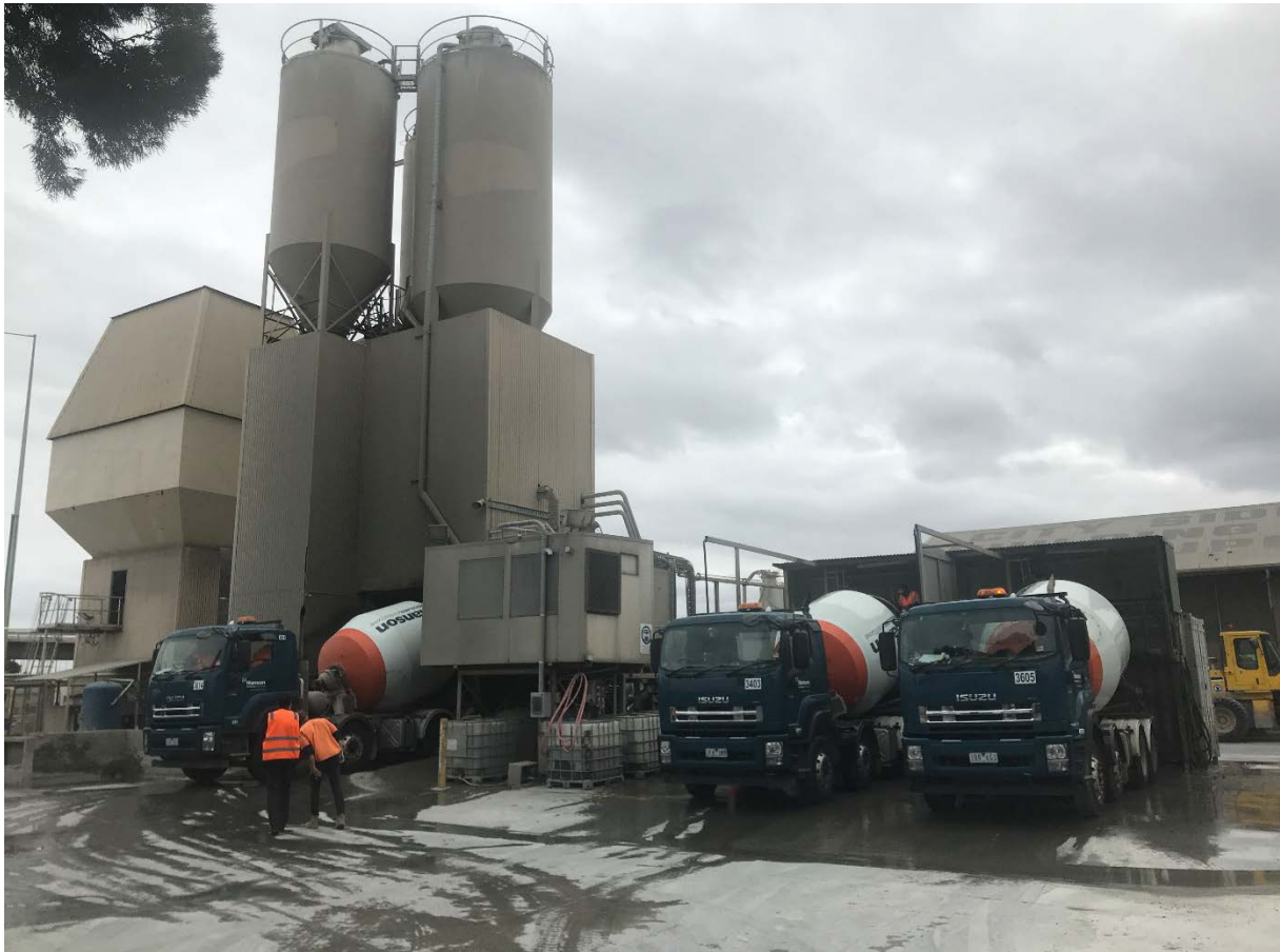
Figure 4 "Sock" and "slump bays" on Hanson site
