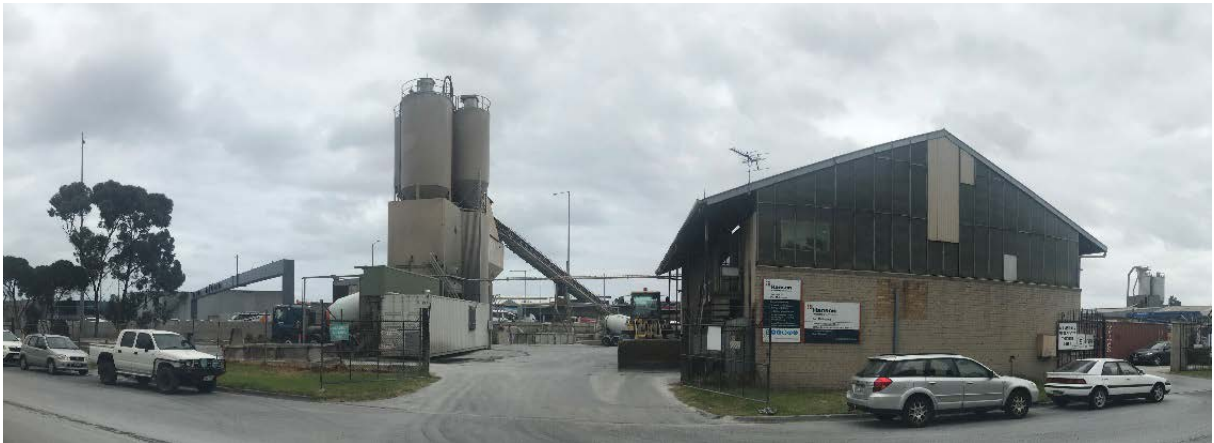
Figure 2 The Hanson site, Boundary Street frontage
