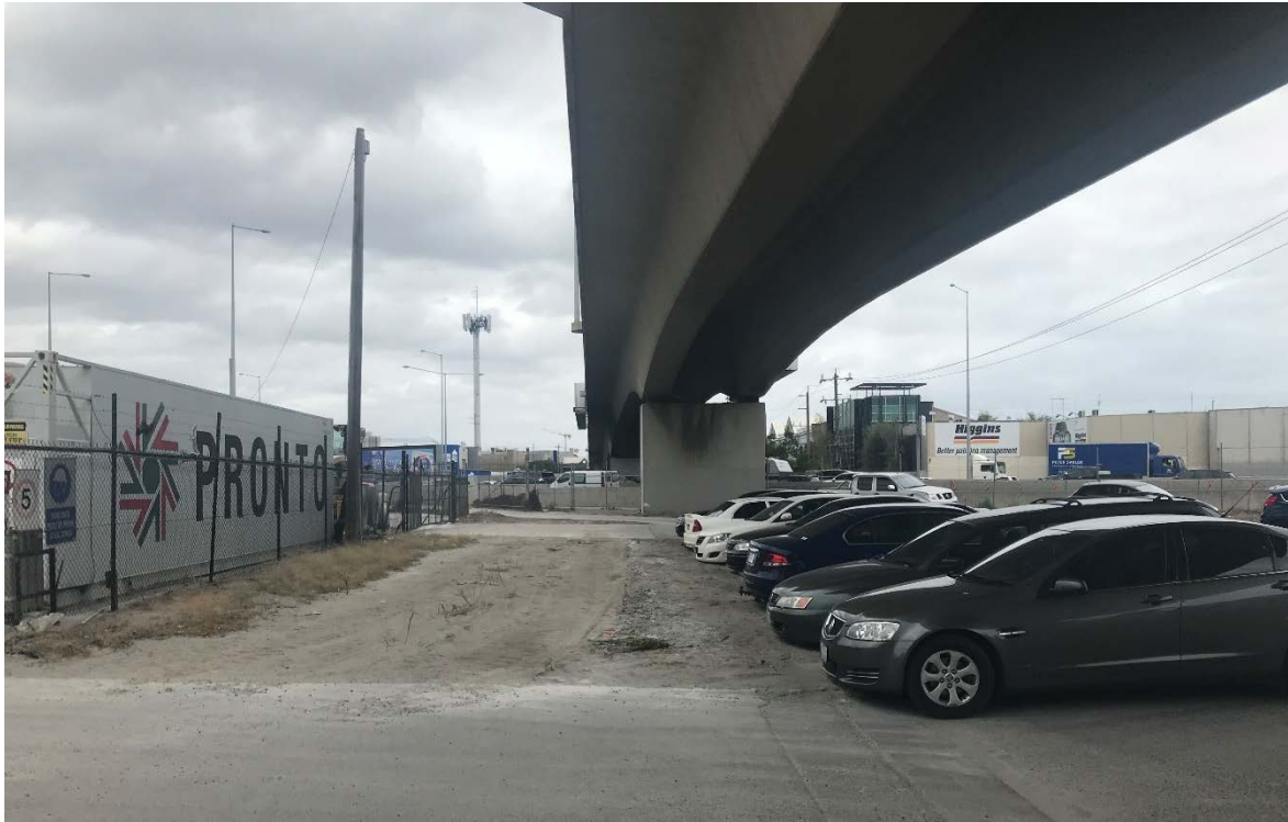
Figure 8 Ingles Street, to the rear of the site
