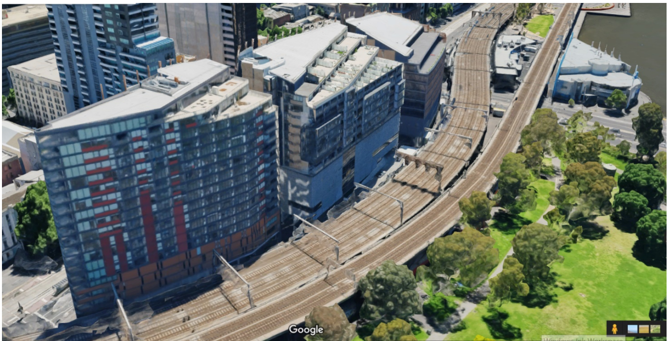
Northbank development in Flinders Street (source: Google Maps)
