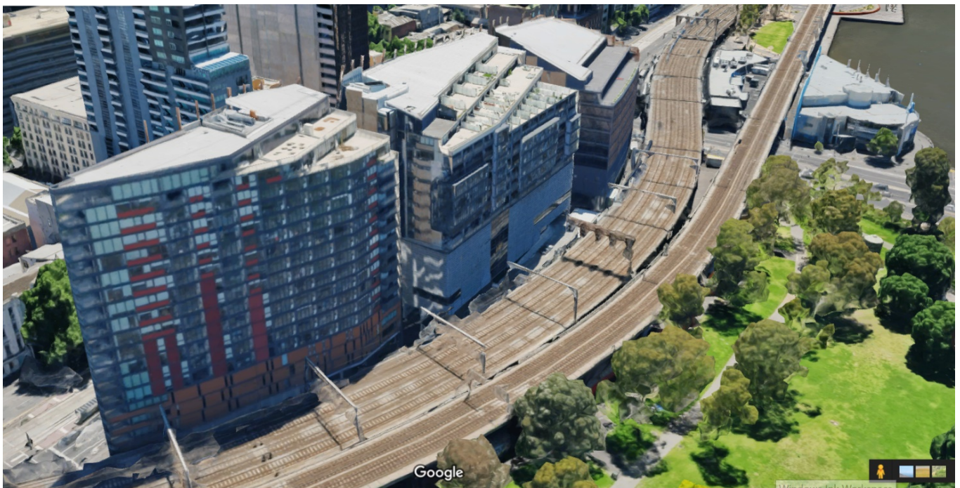
Northbank development in Flinders Street (source: Google Maps)
