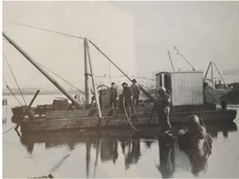
Figure 44: J.W. Lindt photograph that shows workers (some dressed in diving gear) dredging the lower Yarra, below the Falls, c.1886. The punt used for dredging was named the Bunyip (source: Shar Jones, J.W. Lindt: Master photographer, 1985)
