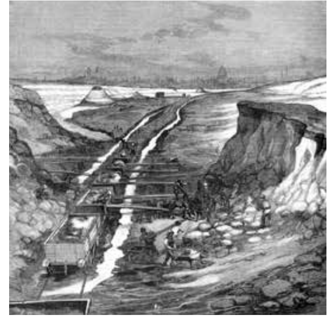
Figure 43: Excavation works at Fishermans Bend, Yarra River, 1880 (source: Pictures Collection, State Library of Victoria)
