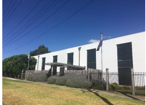
Picture 2 - 162-188 Turner St, site frontage
