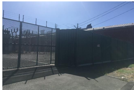
Picture 4 – 90-96 Johnson Street, immediately south of the subject site
