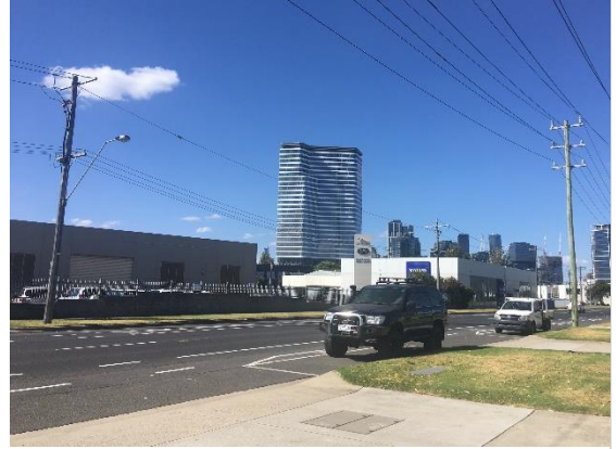
Picture 2 – 351-387 Ingles Street, view from Turner Street
