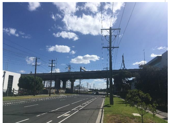
Picture 6 – Turner Street, looking West at City Link elevated bridge.
