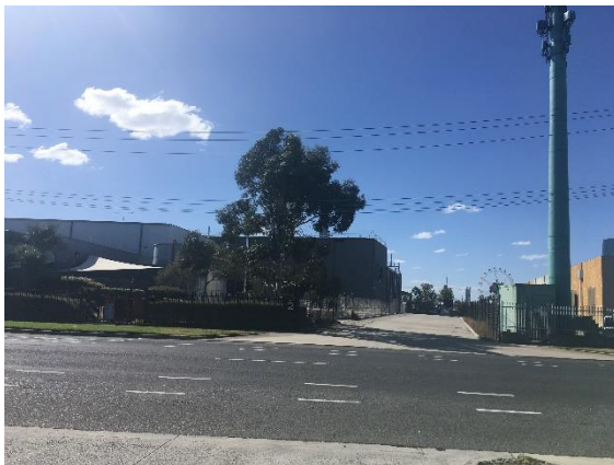
Picture 3 – 161-189 Turner Street, site immediately abutting to the south-west
