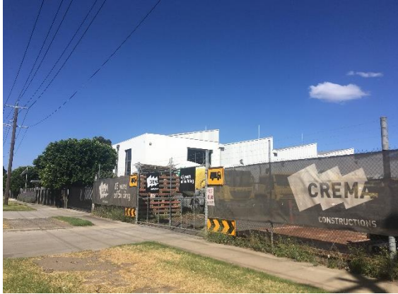
Picture 1 - Looking west, adjacent site 150 Turner St and subject site.
