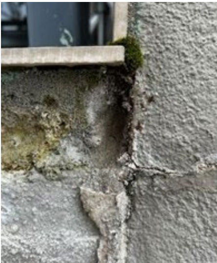
Tiling not sitting flush on concrete slab. No screed or membrane present. Moss and mould evident from pooled water.
