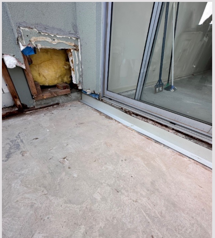
Damaged insulation.
