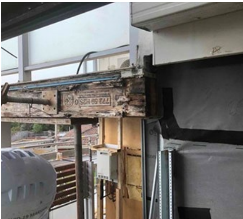
Water ingress to balconies – owners corporation not rectifying as part of the program. MBS has previously issued Emergency Order on these units.
