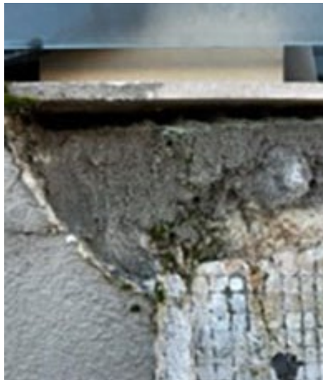
Tiling not sitting flush on concrete slab. No screed or membrane present. Moss and mould evident from pooled water.
