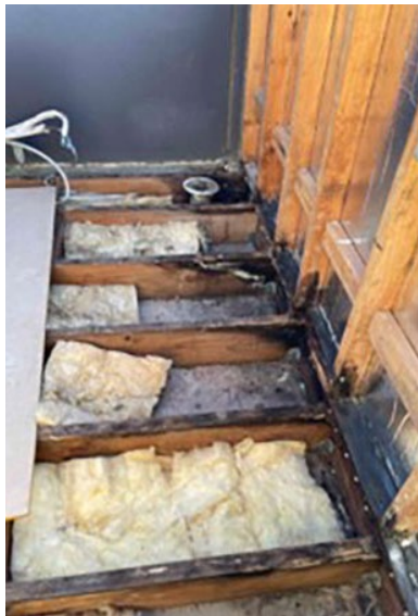
Figure 13. Example of insufficient or no waterproofing affecting a balustrade on a funded building in CSV's program (comprising 12 sole occupancy units)
