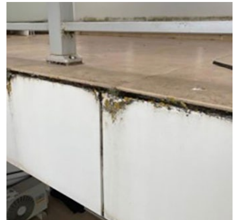
Water ingress to balconies – owners corporation not rectifying as part of the program. MBS has previously issued Emergency Order on these units.
