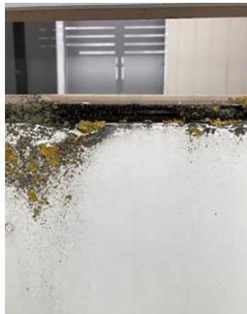
Water ingress to balconies – owners corporation not rectifying as part of the program. MBS has previously issued Emergency Order on these units.
