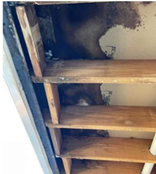
Figure 13. Example of insufficient or no waterproofing affecting a balustrade on a funded building in CSV's program (comprising 12 sole occupancy units)
