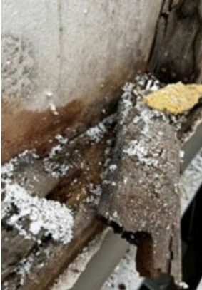
Bottom plate of timber framed balustrade.
