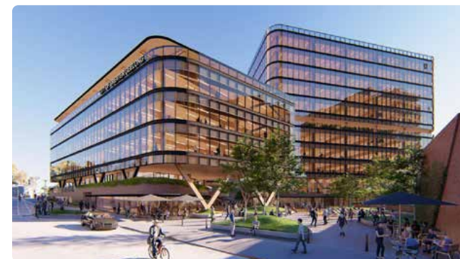
Above: The City of Greater Geelong's new office will achieve the highest standards of sustainable design with a 6 Star Green Star Design and As-Built Rating as well as a 5 Star NABERS Energy Rating.
