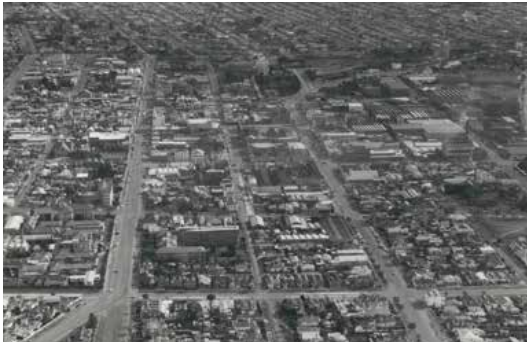
Above: Central Geelong looking west down Ryrie Street circa 1954
