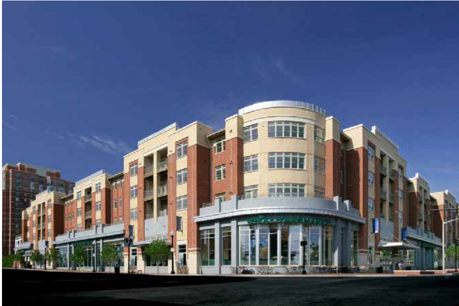
Above: Example artists impression of development on prominent corners providing clear and distinct architectural expression via entrances, windows, canopies, steps, and recesses and projections, should highlight individual elements and reinforce a variety of scales and textures within the podium.
