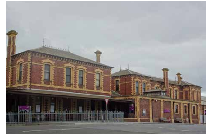
Above: An attractive, safe and high amenity station forecourt is an essential part of the Geelong Station role as a gateway location into Central Geelong. Preserving that amenity while master planning work is progressed is an important part of this Framework Plan.
