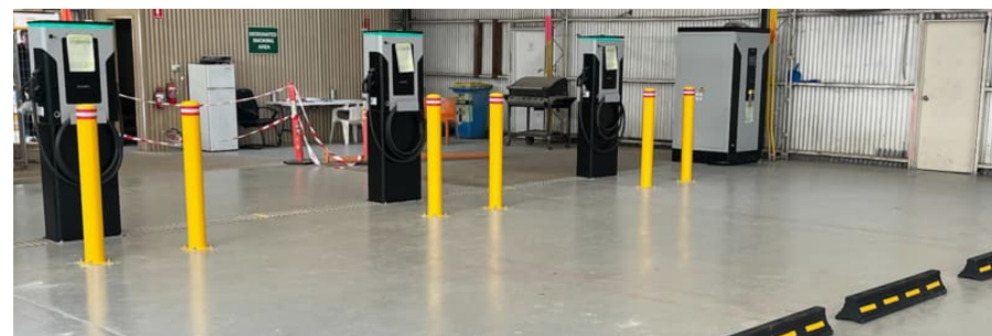
Figure 13 Three charging dispensers installed at Seymour depot, operated within existing 100kW electrical capacity
